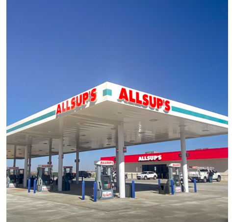
One of Yesway's new Allsup's convenience stores located in New Mexico.
